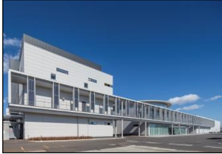
Plant exterior view.
