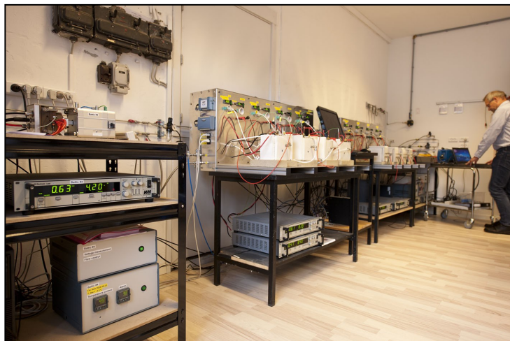
Part of Danish Power Systems' testing facilities.
