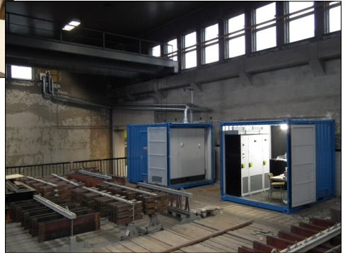
50 kW PEMFC system, run with by-product H 2 from sodium chlorate production, Äetsä, Finland.
